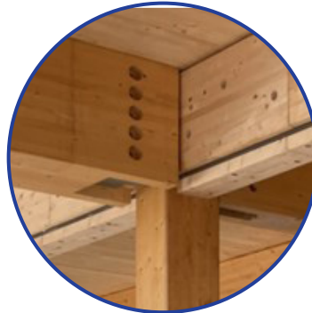
Mass Timber Structure
