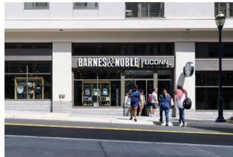
Front Street Lofts Delivered 2015 Hartford, CT
