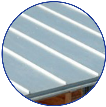
Standing Seam Metal Roofing
