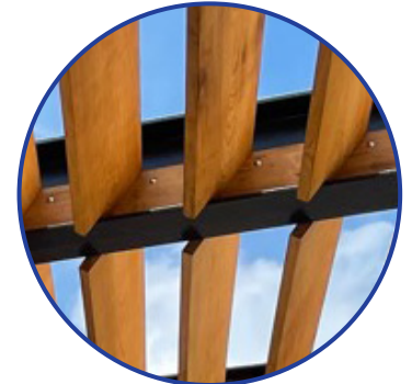
Cedar Slat Roof Framing Shade Structure
